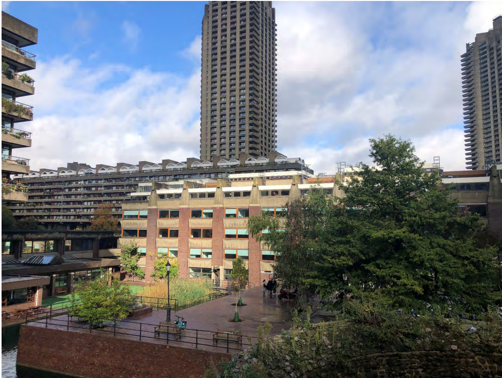
View from Wallside (Figure F)
