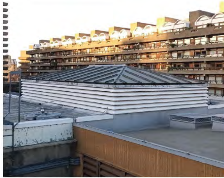
Fig 1: View a of South and East Elevations, looking North West towards Defoe House
